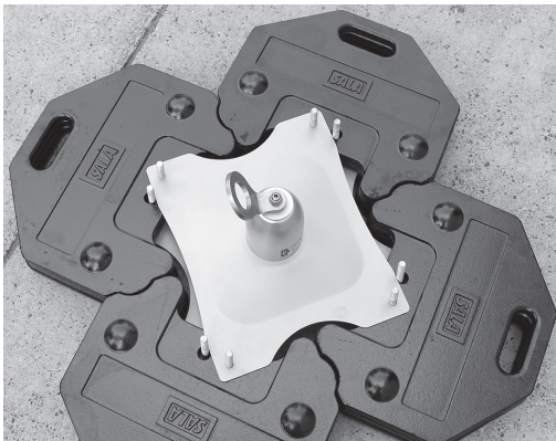
Figure 11 - Place Roof Top Anchor on U-Bolts
