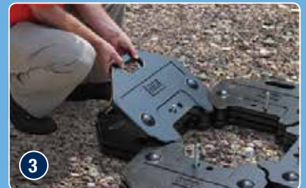
3 Stack plates (weights) over bolts and onto rubberised plates
