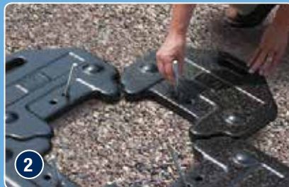
2 Install the "L" bolts into the slots of the rubberised plates
