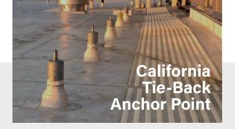
Cal-OSHA mandates special roof tie-backs are installed on every building 36 feet or more in height, and stipulates unique design, system layout, engineering and testing criteria. Guardian has designed custom anchors to meet these requirements. Get in touch for more detailed information.
